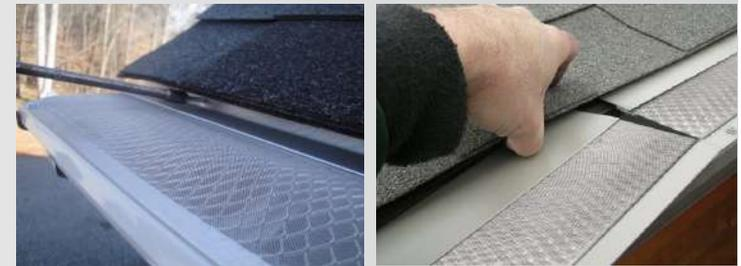
Leaf Solution Xtreme gutter guards can be mounted to the fascia or under the shingle.
